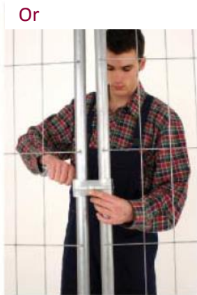
Fix the standard connector with a wrench.
