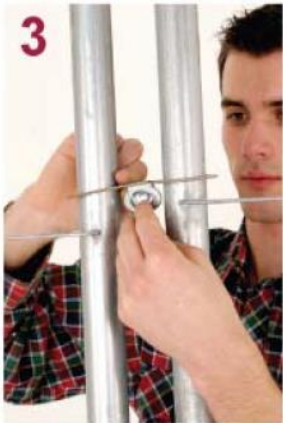
Fix the brackets with screws and nuts.
