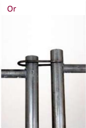
Move the wire loop over the post of the neighboring panel.
