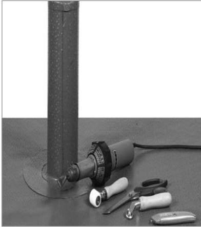
30. Finished covered pipe
