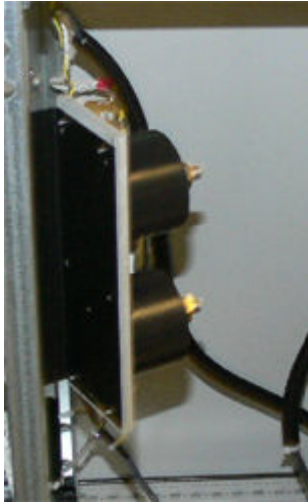
Figure 44: Output Lightning Arrestors
