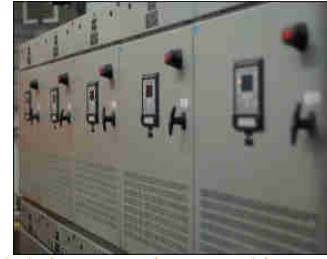
Freedom Series Switchgear Regulators provide constant current to the airfield lighting circuits.
