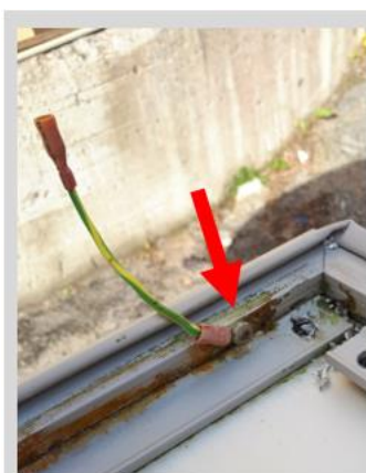
[A] Remove earthing cable
