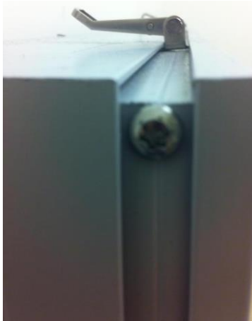
FIGURE 1 - OPEN THE TRACK MARKINGS
