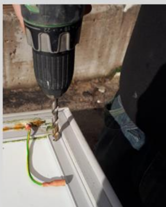
[B] drill a hole on the shorter back list until you reach the underlying rubber
