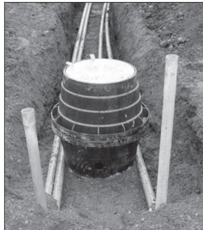
Typical Installation in Back-to-Back Configuration
