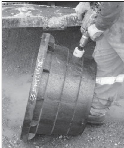
Pullpits are easily drilled to accept cable duct
