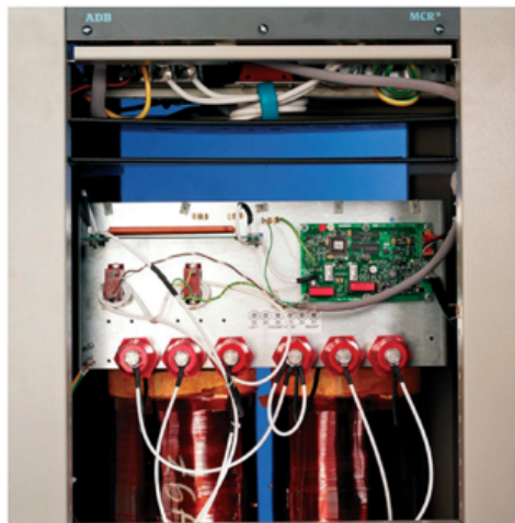
Fig. 11: Taps on secondary of output transformer
