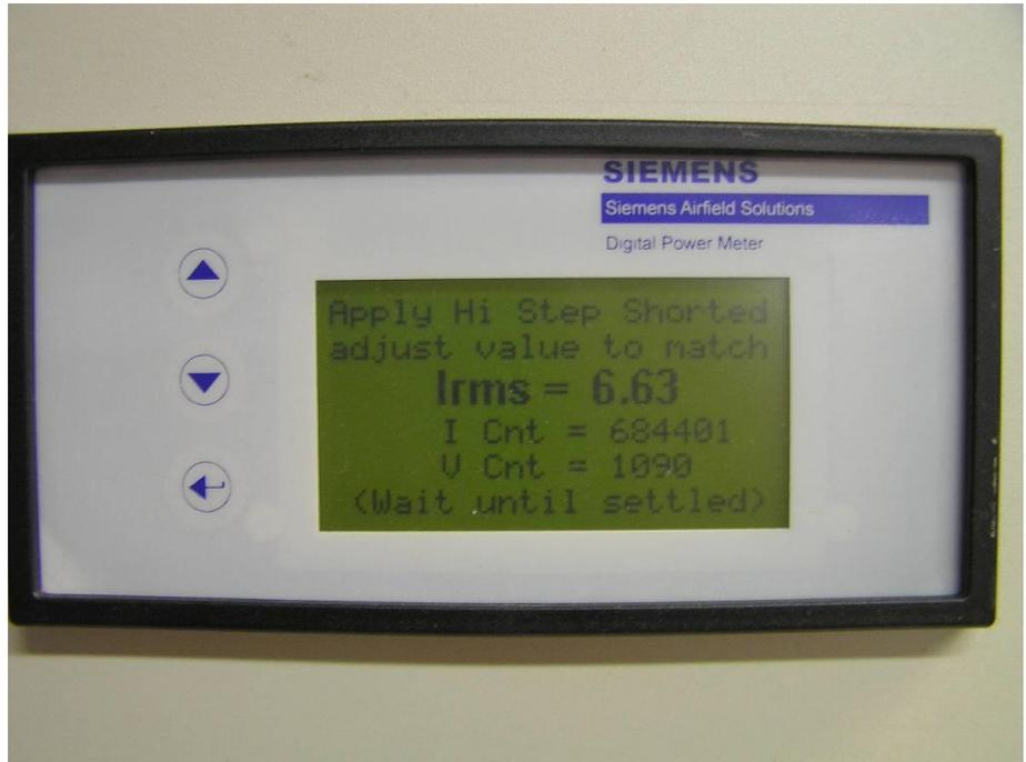
(PIC 4) Follow the instructions on the display, applying the CCR's highest step to a shorted load. Measure the CCR's output current with a current clamp and adjust the DPM display with the UP/DOWN buttons so the Irms value matches. Wait until the CNT values on the display settle and press <.
