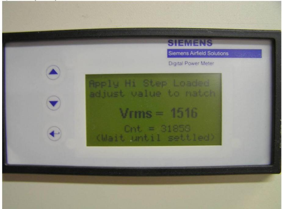
(PIC 8) Follow the instructions on the display, applying the CCR’s highest step to the field load. The CCR’s output voltage can be measured with an AC voltage meter at the secondary of the Output Voltage Feedback Transformer. This voltage may be found on the terminal block at the bottom of a SGRS cabinet. Adjust the DPM display with the UP/DOWN buttons so the Vrms value matches. Wait until the CNT values on the display settle and press <.
