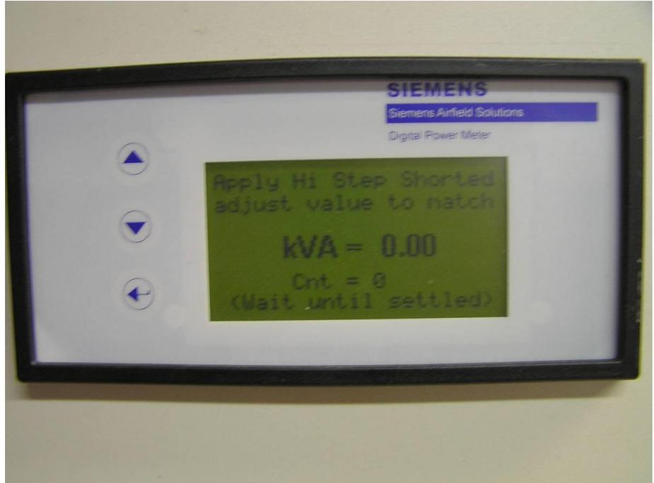
Follow the instructions on the display, applying the CCR's highest step to a shorted load. The CCR's VA at this point should be zero. Adjust the DPM display with the UP/DOWN buttons so the VA value reads zero. Wait until the CNT values on the
