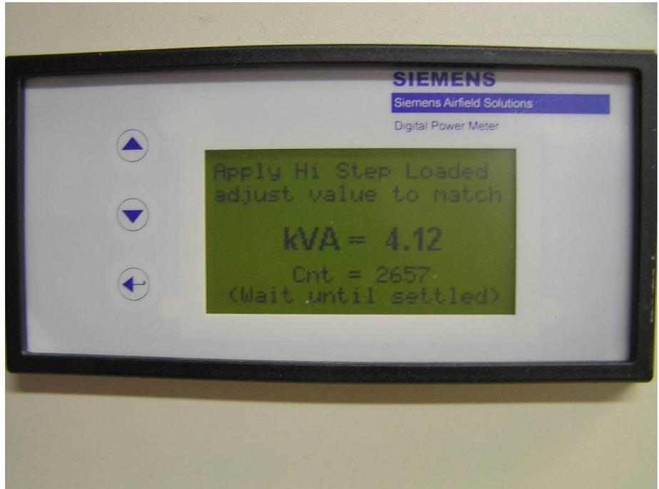
(PIC 12) Follow the instructions on the display, applying the CCR's highest step to the field load. The CCR's VA can be calculated by multiplying it's output current and voltage values together. Adjust the DPM display with the UP/DOWN buttons so the VA value matches your calculated value. Wait until the CNT values on the display settle and press <.
