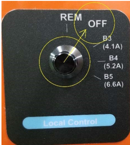
Figure 12: Remote/ Local Switch in the OFF position
