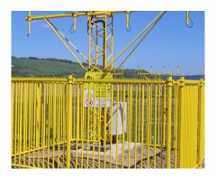
Exel frangible fences are transparent to electromagnetic signals, easy to install and practically maintenance free.
