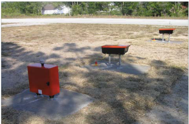
Fig. 1 Style A L-881 (2 Box) PAPI System
