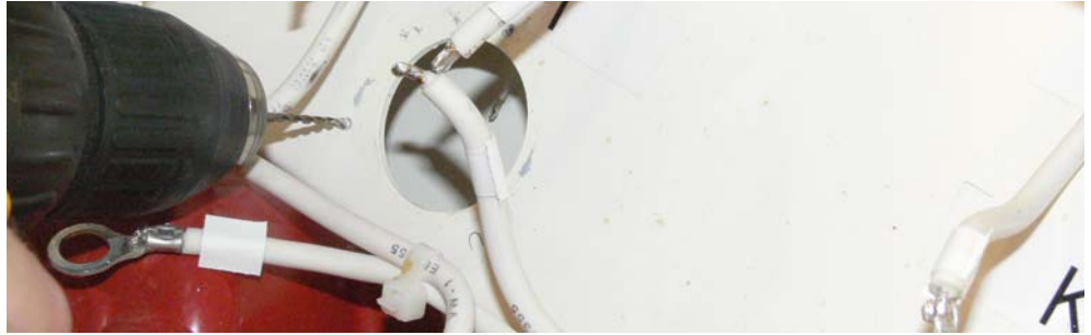
Figure 11: Drilling the pilot holes
