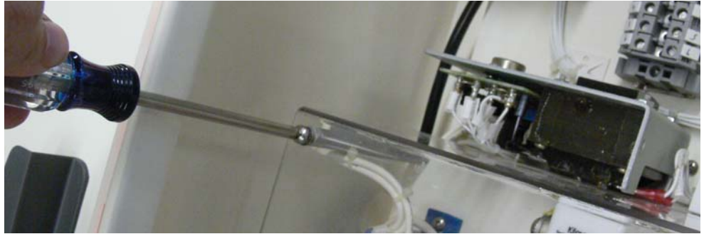
Figure 21: Installing the safety shield
