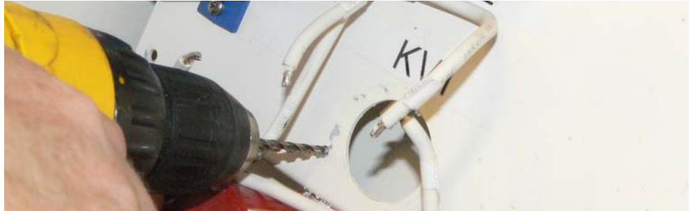
Figure 12: Drilling the holes for the screws
