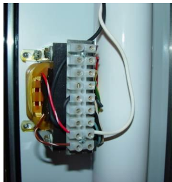
Figure 2: Power Supply Transformer to Remove
