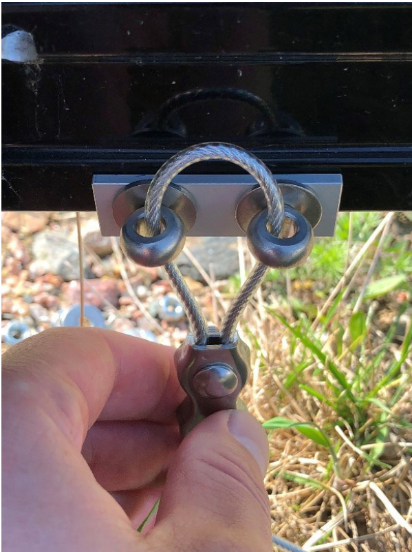
Figure 12: Mount washers and eye bolts
