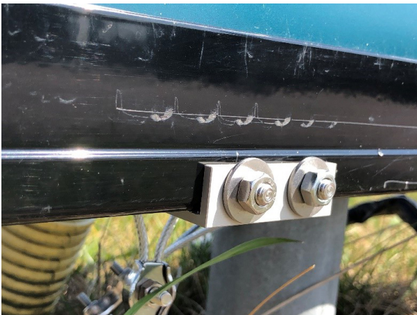
Figure 16: Mount washers and lock nuts
