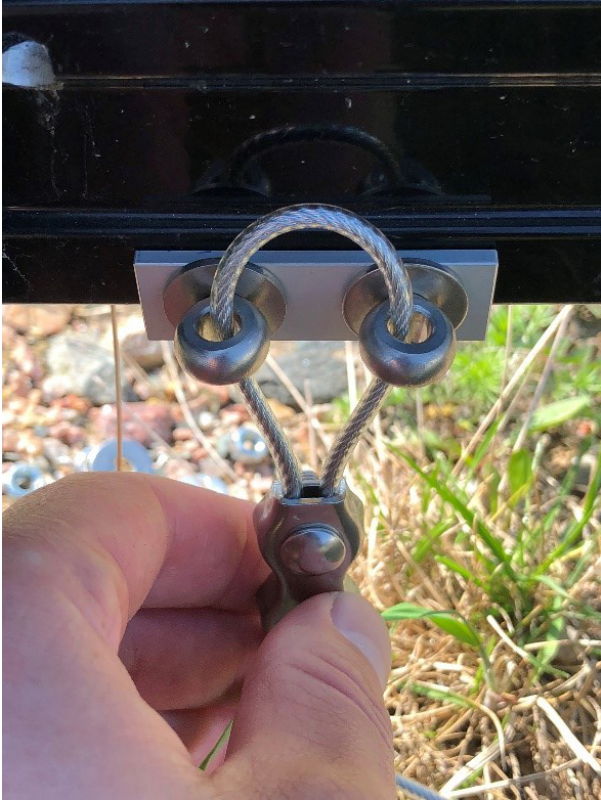
Figure 15: Mount washers and eye bolts
