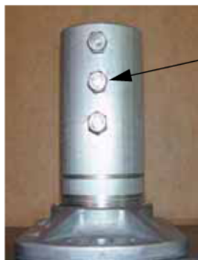
Figure 5: Sign Frangible Coupling
