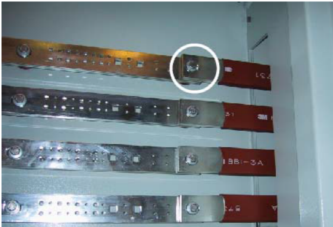
Figure 12: Bus Bar Installation Between Cabinets
