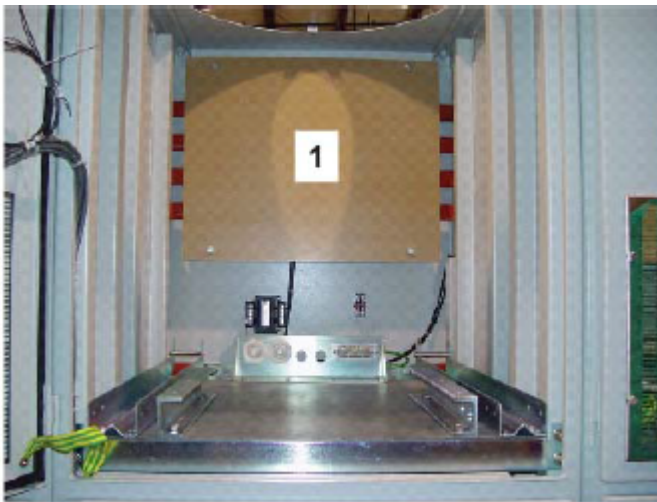
Figure 19: Glastic Shield Stand-Offs
