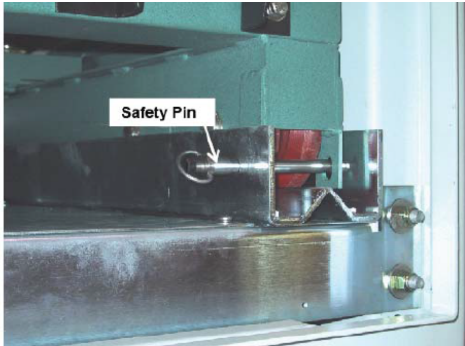
Figure 39: Securing Powerpack in Enclosure Bay
