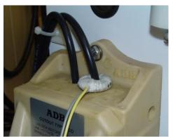
Fig 8 Installation of Current Feed Back Transformer
