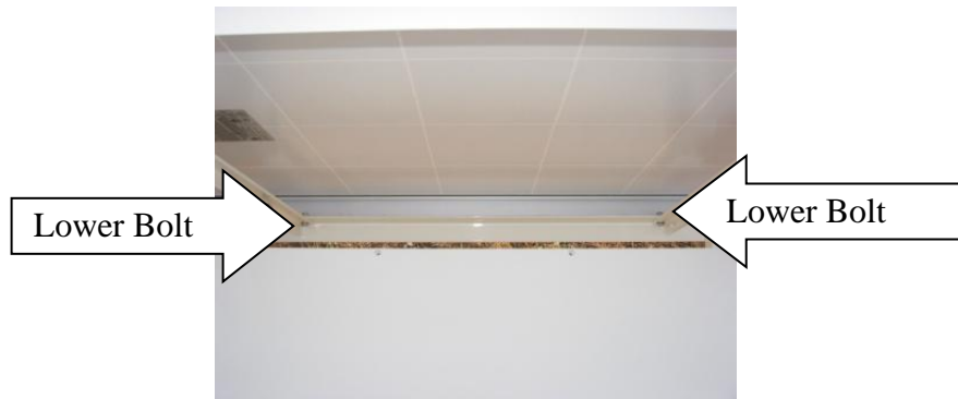
Figure 9. Lower Solar Panel Mounting Bolts
