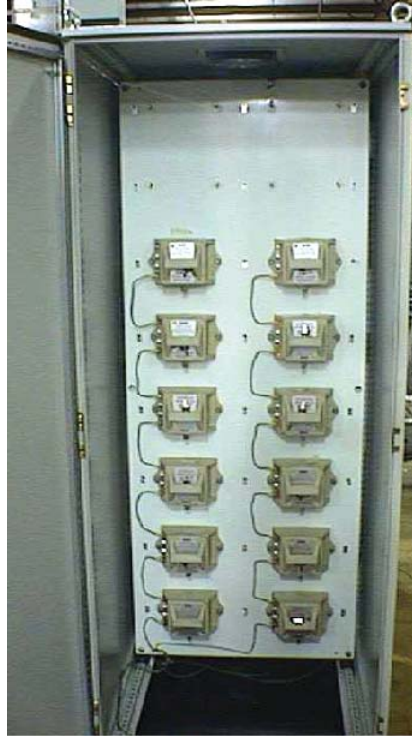
Figure 6: S1 Series Circuit Cutout Bay
