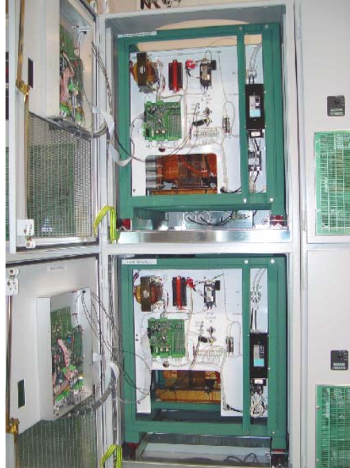
Figure 11: Powerpacks inserted into Bay
