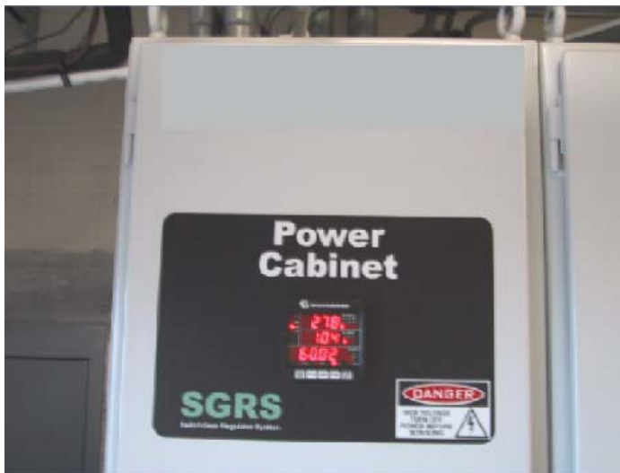
Figure 3: Digital Voltage and Current Meter
