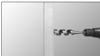
Bor 32mm hull i stender.
